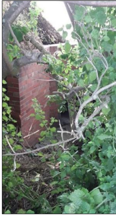
View 4: Brickwork headwall
