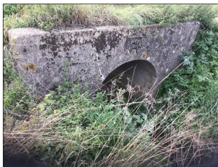
View 6: Golden Bridge Sewer (ref. G)
