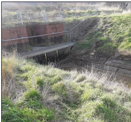
View 5: South-west view showing the upstream face of Bowaters Sluice.
