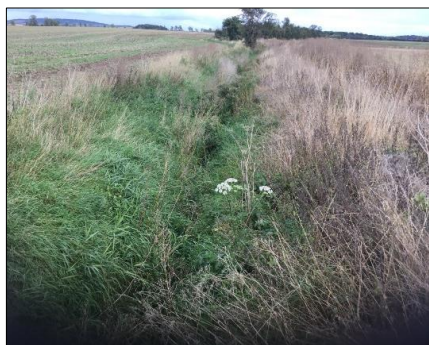
View 5: Golden Bridge Sewer (ref. G)
