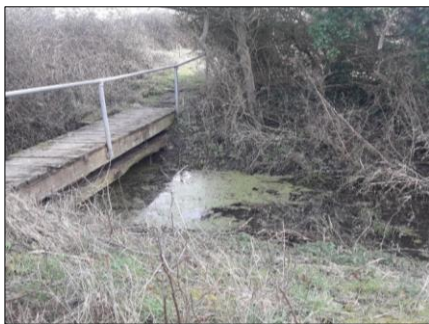
View 3: Orsett Fen Sewer (ref. F)
